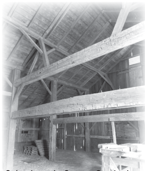
Swing beam in Sayer – Stander barn measures 10" X 17". Canted queenpost with a strut supports purlin.
