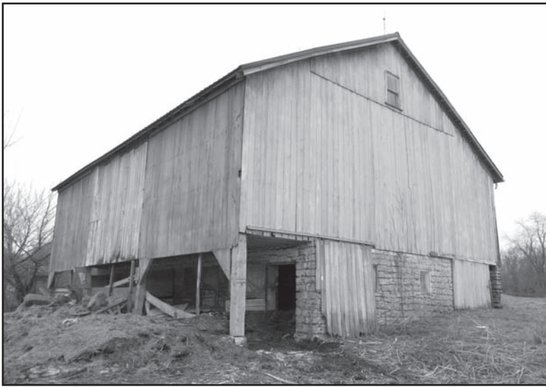
Left: Elliot – Smiley barn with a posted forebay and limestone basement, circa 11850's, is constructed entirely of sawn timber from a mill that formerly stood on the property.
