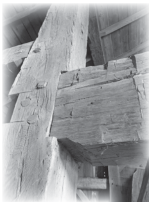
Right: Hand hewn timbers in Sayer – Stander barn are sup- ported by sawn bracing, includ- ing this one with irregular sides.
