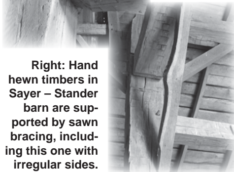
Swing beam in Sayer – Stander barn measures 10" X 17". Canted queenpost with a strut supports purlin.
