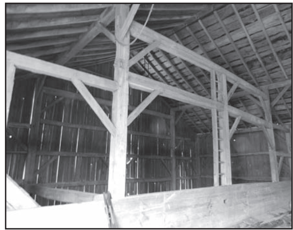
Left: Elliot – Smiley barn with a posted forebay and limestone basement, circa 11850's, is constructed entirely of sawn timber from a mill that formerly stood on the property.
